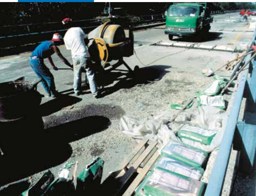
Reforming road joints
