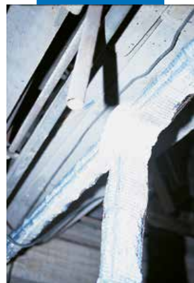
Deteriorated concrete structure
