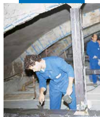
Pouring Mapegrout Hi-Flow into metal formwork
