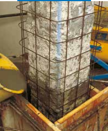
Pouring into a formwork
