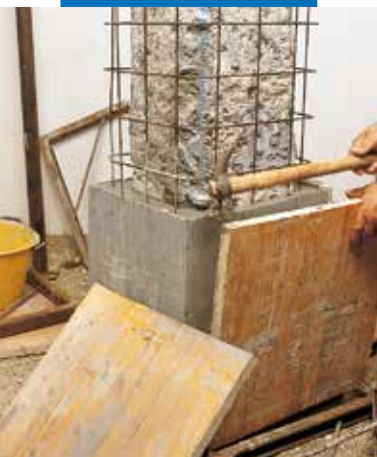
Removing wooden formwork
