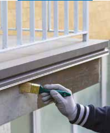
Application of Planiseal WR 40 by brush
