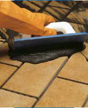
Grouting an external klinker tile floor with Keracolor GG mixed with Fugolastic
