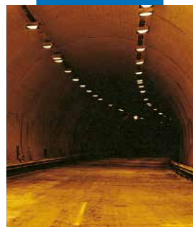
Application of white Planiseal 88 by spray gun in highway tunnel
