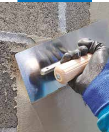
Application of Planiseal 88 by trowel
