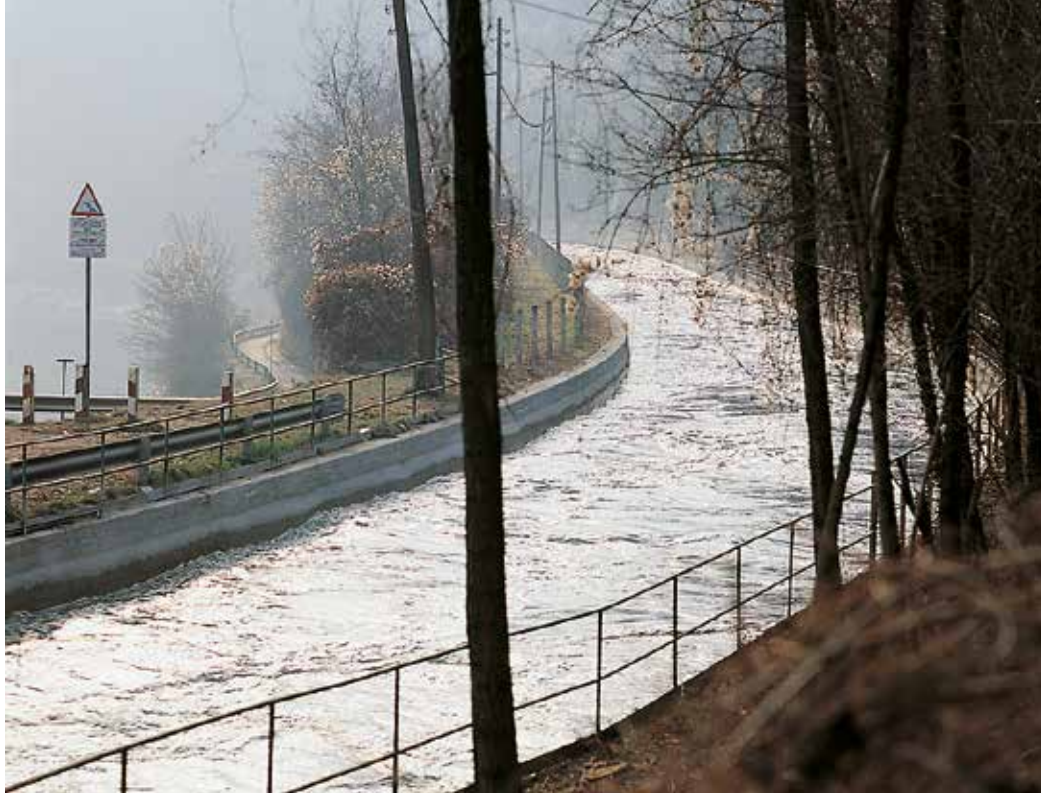
Bertini hydroelectric canal - Como - Italy. Surfaces treated with Planiseal 88
